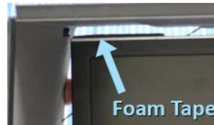
Image 4 Foam Tape Placement
